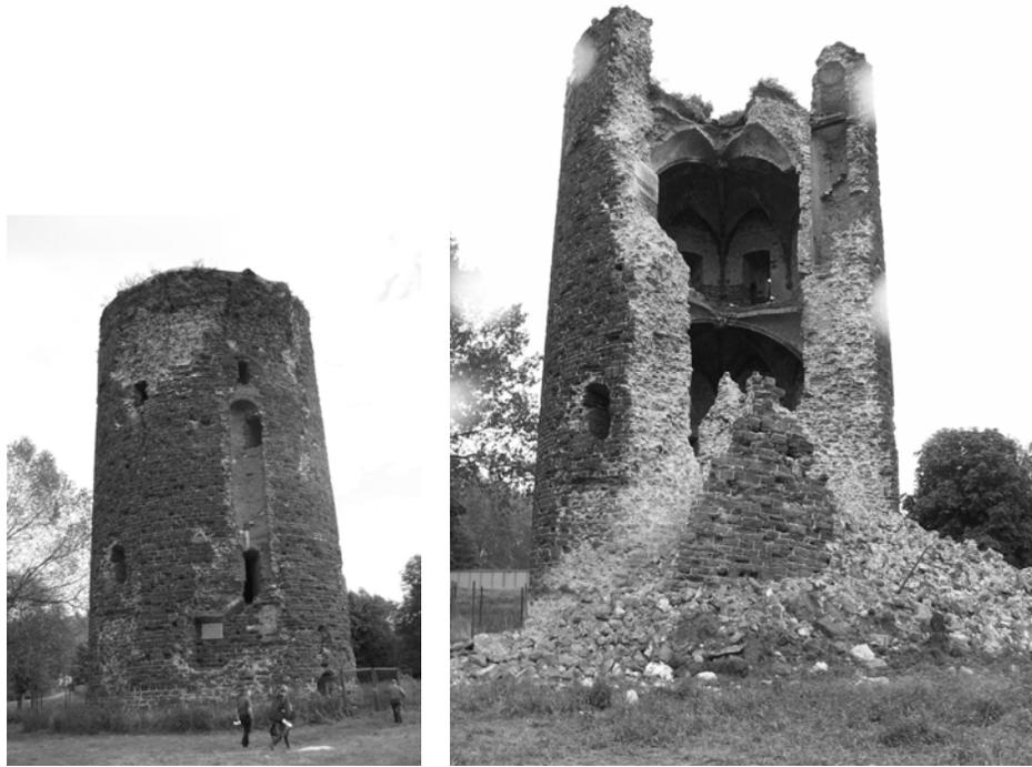
Fig. 1. Maagden tower at Zichem, Belgium, before and after collapse (June 2006)
